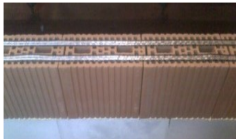
Figure 3 – Armature de joint horizontal
